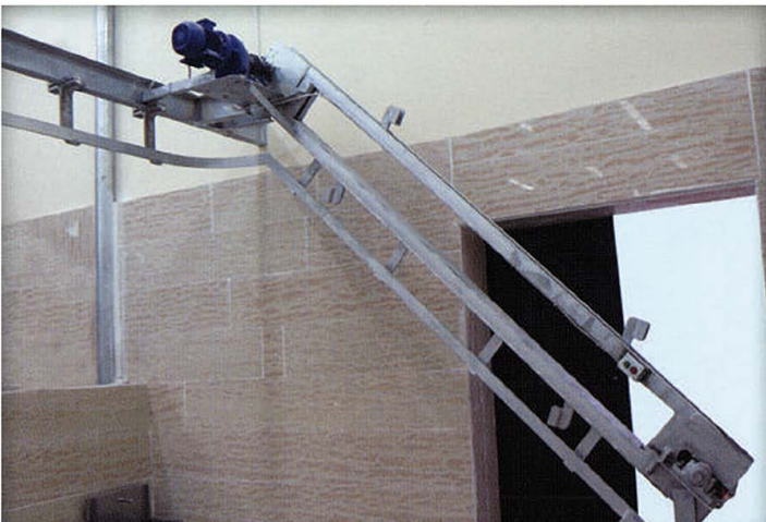
SHEEP LIFTING ELEVATOR
