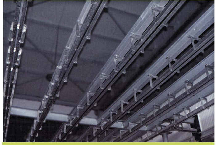
TWIN RAIL LINE
